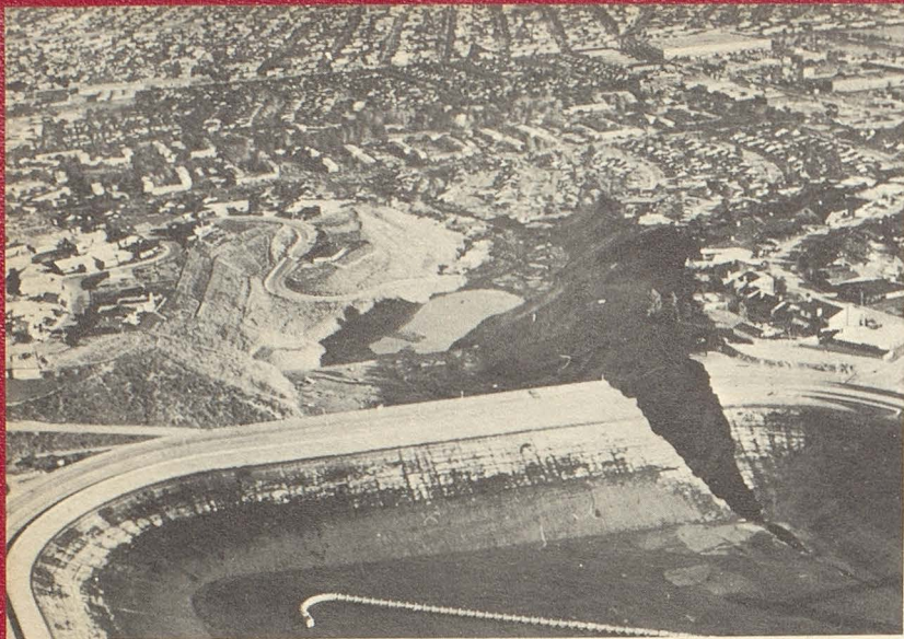
In Los Angeles, Baldwin Hill Reservoir cracked, then broke releasing a torrent which wrecked hundreds of evacuated homes, but produced few casualties.
